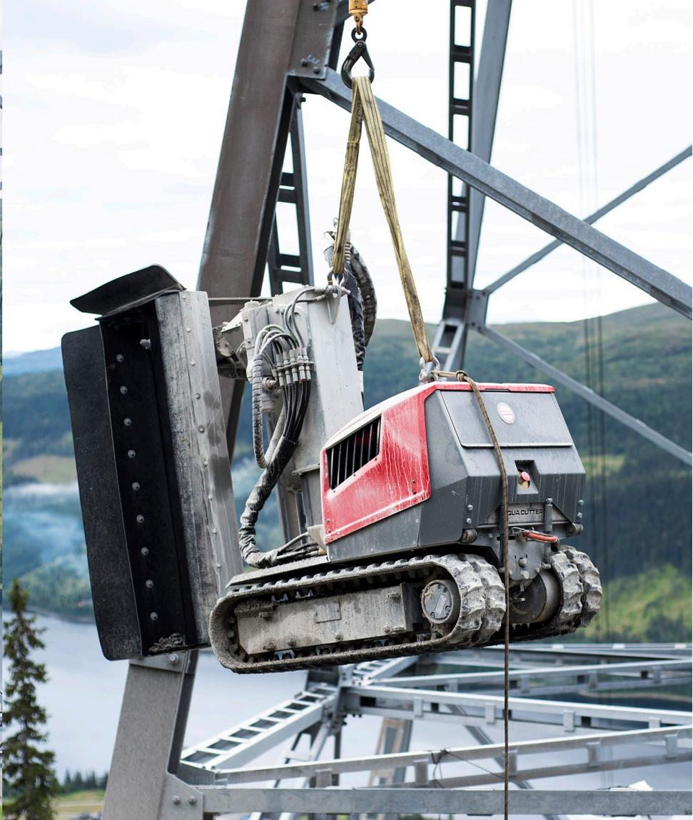
An Aqua Cutter 410A, a remote controlled machine specially designed for applications in confined and inaccessible areas, is being used on the concrete foundation blocks.
