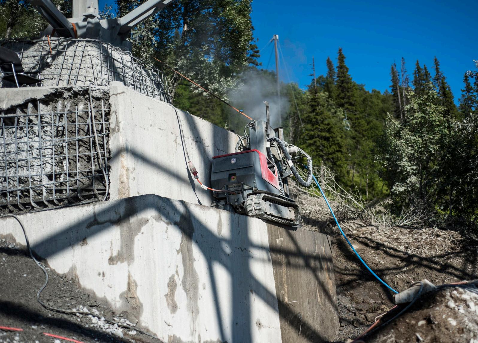
and the pylons. With the hydrodemolition technique it was possible to keep the cableway open during the complete restoration.”
